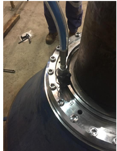
Hydraulic hose connected
