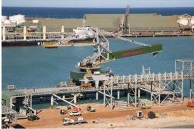
*Loader operations at the \$200 million Geraldton Port facility, which consist of a 300m storage facility, a dedicated berth and the 5000 tph loader.*
