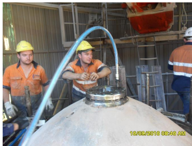
Connect the Pump for Release
