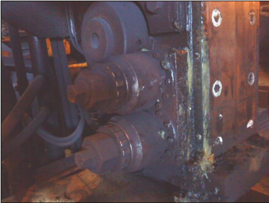
New system installed and in operation
