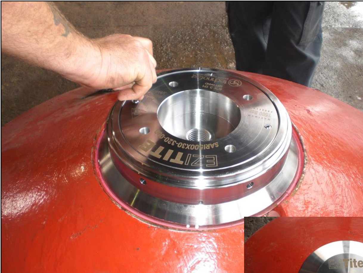
EziTite® Hydraulic Head Nut installed before sacrificial cover is installed.
