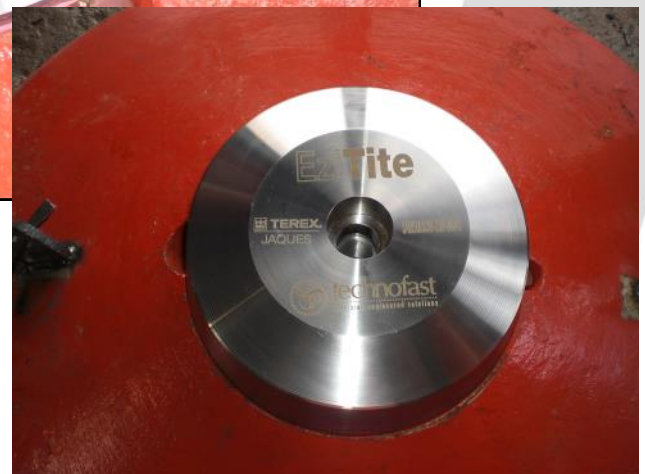
Sacrificial cover installed and the unit is now ready for service.
