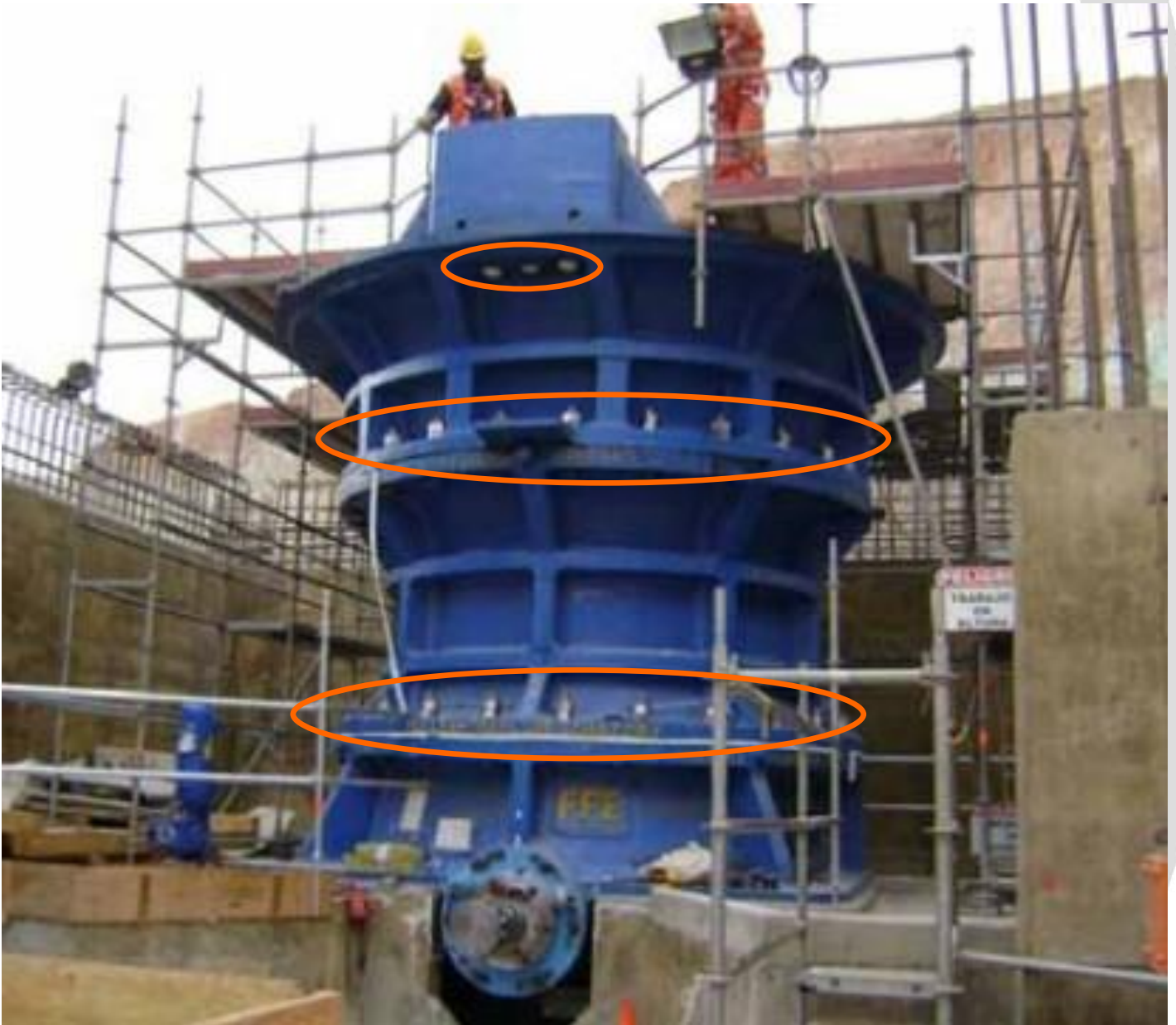
EziTite® Hydraulic Nuts installed prior to commissioning of new crusher..
