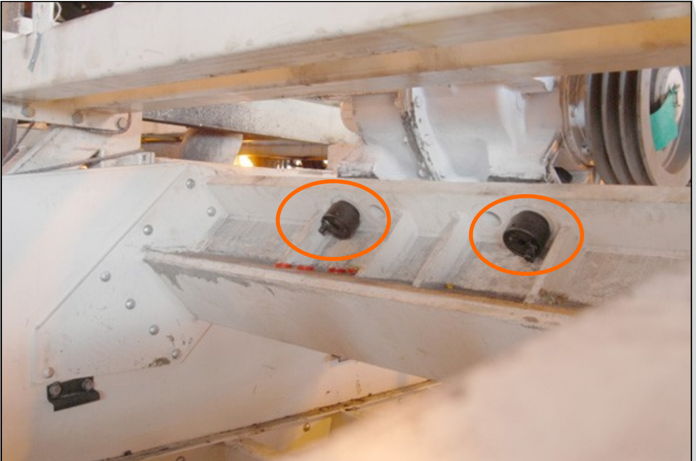
EziTite ® Hydraulic Bolts installed to secure exciter motors ready for service.
